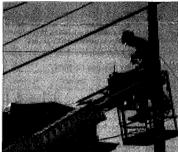
ABOVE: A worker in a bucket boom checks the splice on a Q-Life fiber optic cable
